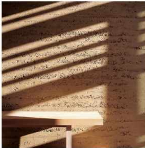
© Lehm Ton Erde; Lehmmauer Vigilius Mountain Resort (Matteo Thun / Martin Rauch)
